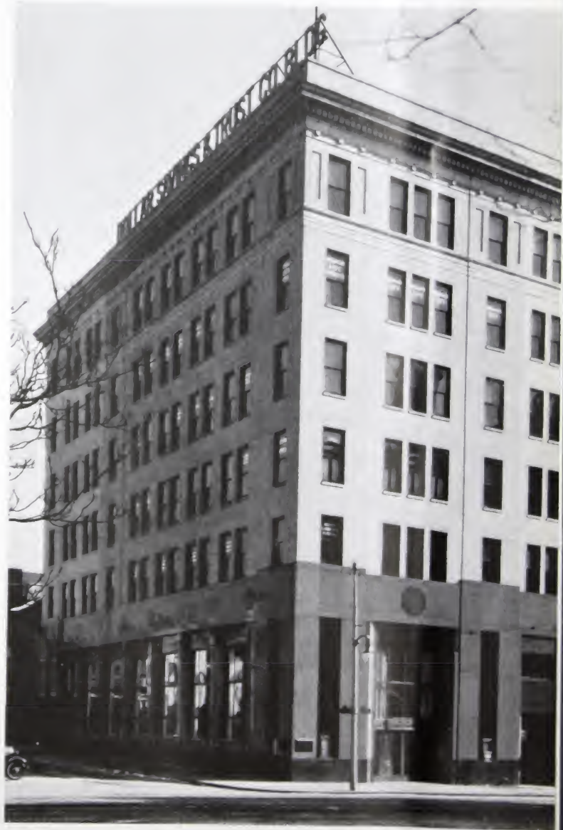
Dollar Savings & Trust Company Building Press C. Dowler, Architect D. T. Riffle, Pittsburgh, Pa., Contractor Hillside Stone & Supply Co., Pittsburgh Medusa Waterproofed Gray Portland Cement used in all the brick mortar.
